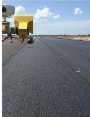
*The PAVE-IR Scan's scanner records the asphalt temperature over the entire width of the paved surface*
