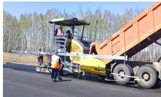
The Big Sonic-Ski with its four sensors achieves the highest levels of planarity when resurfacing the road link from Irkutsk to Taishet
