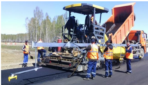
The Big Sonic-Ski with its four sensors achieves the highest levels of planarity when resurfacing the road link from Irkutsk to Taishet
